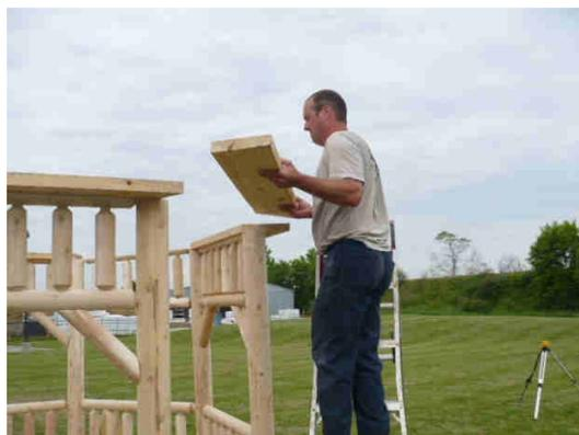
**Step 6.** With your top plate installed and secure, you will now install the fascia boards and rafters. The fascia has a mark on the back side. This mark is at the top of the plate on the inside of gazebo. The double rafters are installed exactly over the posts and plate joints. Secure using 2 long screws, at the bottom only for now.
