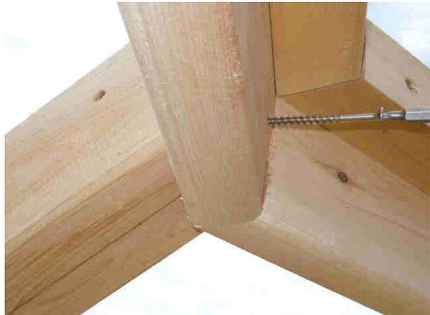
**Step 8.** With the rafters properly secured at the top and bottom, you will now be ready to install the eight pre-shingled roof sections. Carefully lift each section onto the rafters, and secure with three long screws on either side. We supply the galvanized eave starter (drip stop) which you need to cut to the proper length and install at the bottom. Lift the shingles and secure with short nails or screws.
