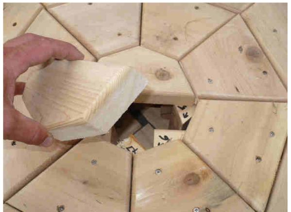
**Step 4.** Now you are ready to install the 4 pre-built gazebo walls. Insert them into the outside circle where marked. If you are assembling a log gazebo you do not want to bolt these just yet, as you need the movement to insert the remaining railing pieces. If this is not a log gazebo you can bolt these together now.
