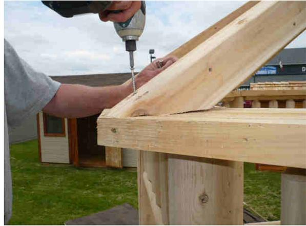
**Step 7.** In this example we are installing a gazebo with a double roof (2 tier roof with cupola). If your gazebo has a double roof you now install the bottom frame for the double roof at the top and screw the frame into the rafter. Use 2 long screws for each rafter. If you do not have a double roof your rafters will come together with a small block at the very top.
