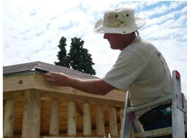
**Step 9.** The next step is to install the angled braces around the bottom in the gazebo. After that, you are ready to lift the cupola onto the gazebo roof. In the photo we show a ladder secured at the scaffold to do this. Be sure to have 2 or 3 people handy when doing this. Slide it into place and screw from underneath into the frame with long screws provided.
