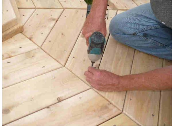
**Step 3.** It is very important to have your floor perfectly level and solid before moving on with the assembly. If it is on a concrete pad this should be taken care of. If it is on patio stones you may need to do some shimming at the posts to get it level. Once your floor is level and solid you also want to fill in the hole in the center. Use 3" stainless screws provided.
