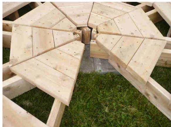
**Step 2.** After you have the 8 floor sections matching up perfectly with each other, you need to bolt them together at the inside circle only. After you have the 8 bolts at the inner circle tight, you can then install the floor boards for this ring as well.
