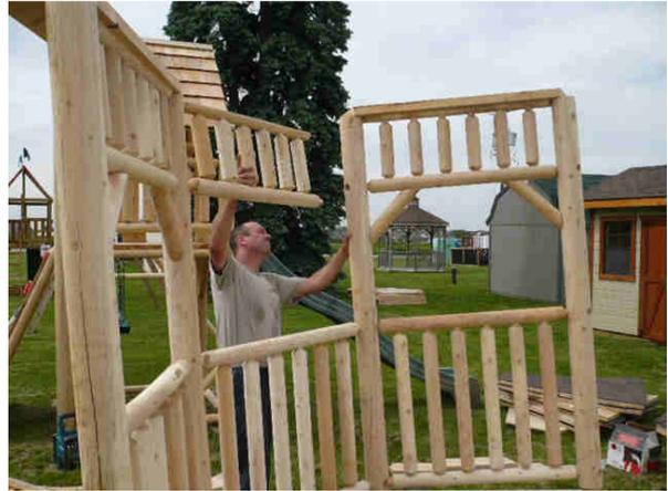
**Step 5.** After you have all railing sections installed and the posts bolted at the bottom, you need to complete the outer ring of floor boards as well. You should have four wide pieces as well to complete the rafter base frame. Install these using long screws and screwing down from the top.
